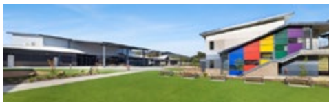
St Matthews Catholic School Mudgee - Secondary Campus
